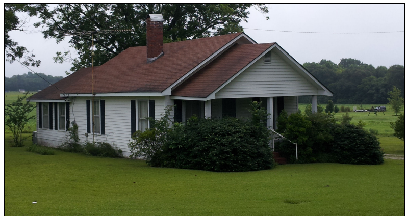
The Peele Home Place, built 1927, kitchen added in 1941.
